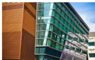
DAVIS HALL ELECTRICAL ENGINEERING CLEANROOM
